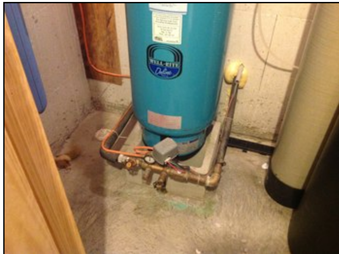
9. Front of the basement
